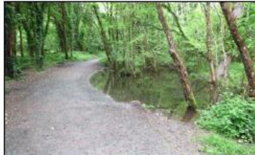
Seepage beside path near first (south) wooden bridge in Knocksink Wood.
