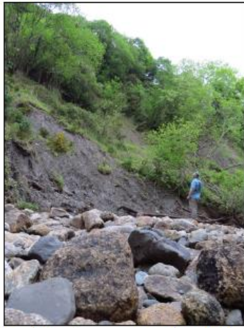
Slope failure (mass movement) on NE bank of river (north of second bridge in Knocksink Wood). Low river flow conditions.
