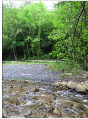
Stone reinforcements on NE riverbank river (between two wooden bridges in Knocksink Wood).
